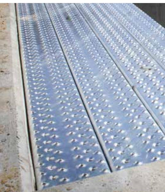
To ensure maximum safety, PcP has designed a cost-efficient solution requiring a little to no maintenance, a smaller pit and 100 % reliability regarding design criteria. PcP's LHD® Low Hole Density gratings are welded together to minimise the level of air flow combined with excellent drainage to ensure any flame extinguishment. In addition, PcP LHD® welded gratings are easy to replace. Each solution is carefully designed and customised to meet your safety requirements and design criteria.
